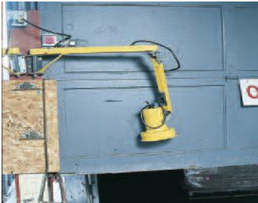
Old technology truck lights are prone to damage from overhead doors and fork lifts.
